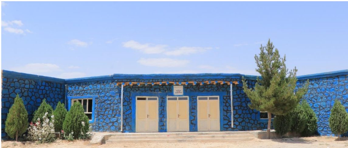
Figure 25 The building of Agho Jan school after rehabilitation.
