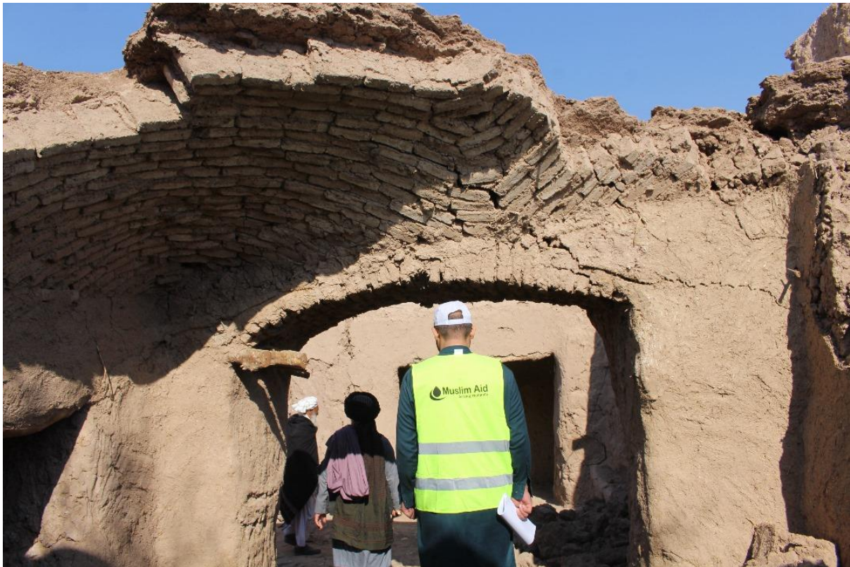
Figure 54 Needs assessment in earthquake-affected areas.
