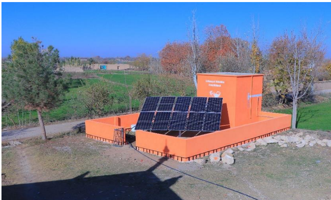
Figure 2 The SPWCs are powered by Solar Panels
