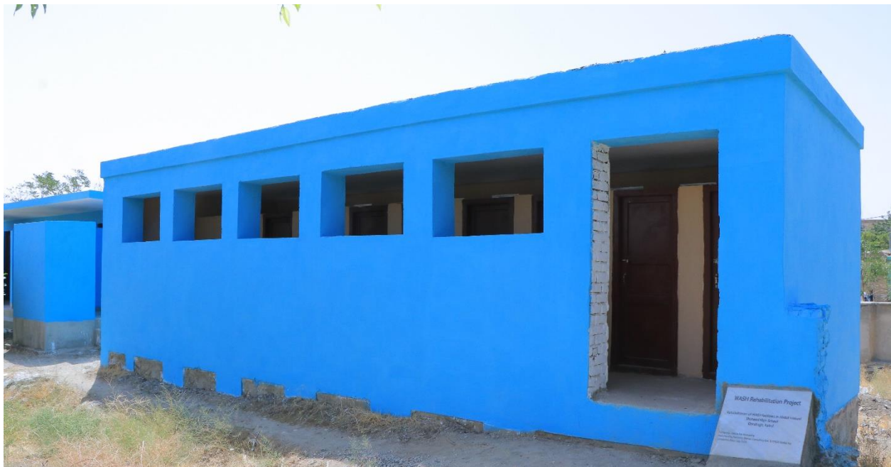
Figure 5 The latrines were extensively rehabilitated in the target schools.
