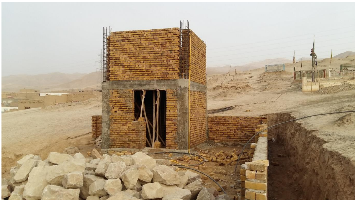
Figure 48 Construction of SPWCs in one of the target villages.
