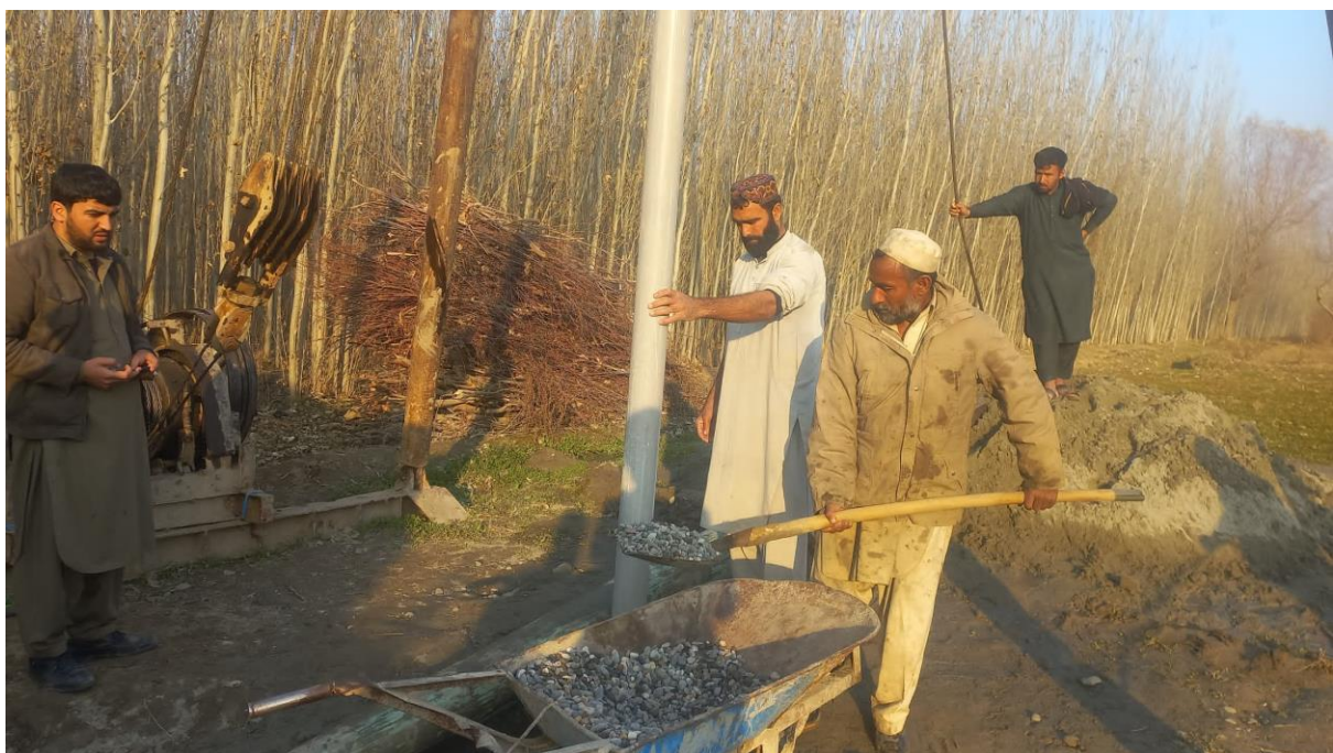
Figure 49 Construction of well in progress.
